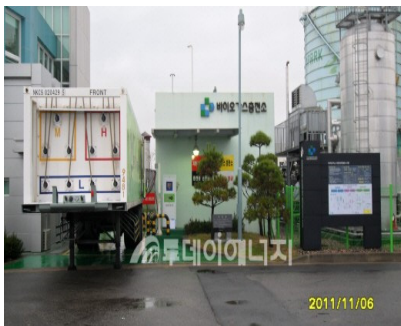
Fig. 3 Biomethane Charging Station
