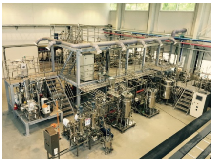
Fig. 4 Biobutanol Pilot Plant
