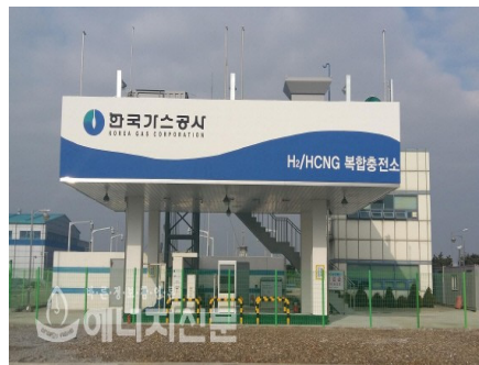
Fig. 2 KOGAS H 2 /HCNG Station
